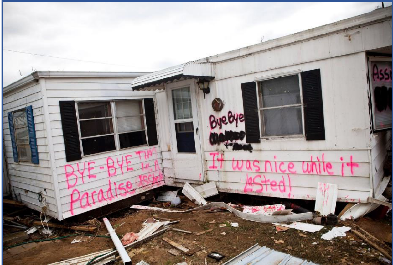
Home damaged by Hurricane Sandy in Highlands, New Jersey (2012).
