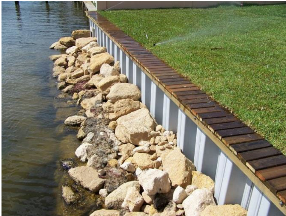
Figure 3-10: Example of bulkhead
