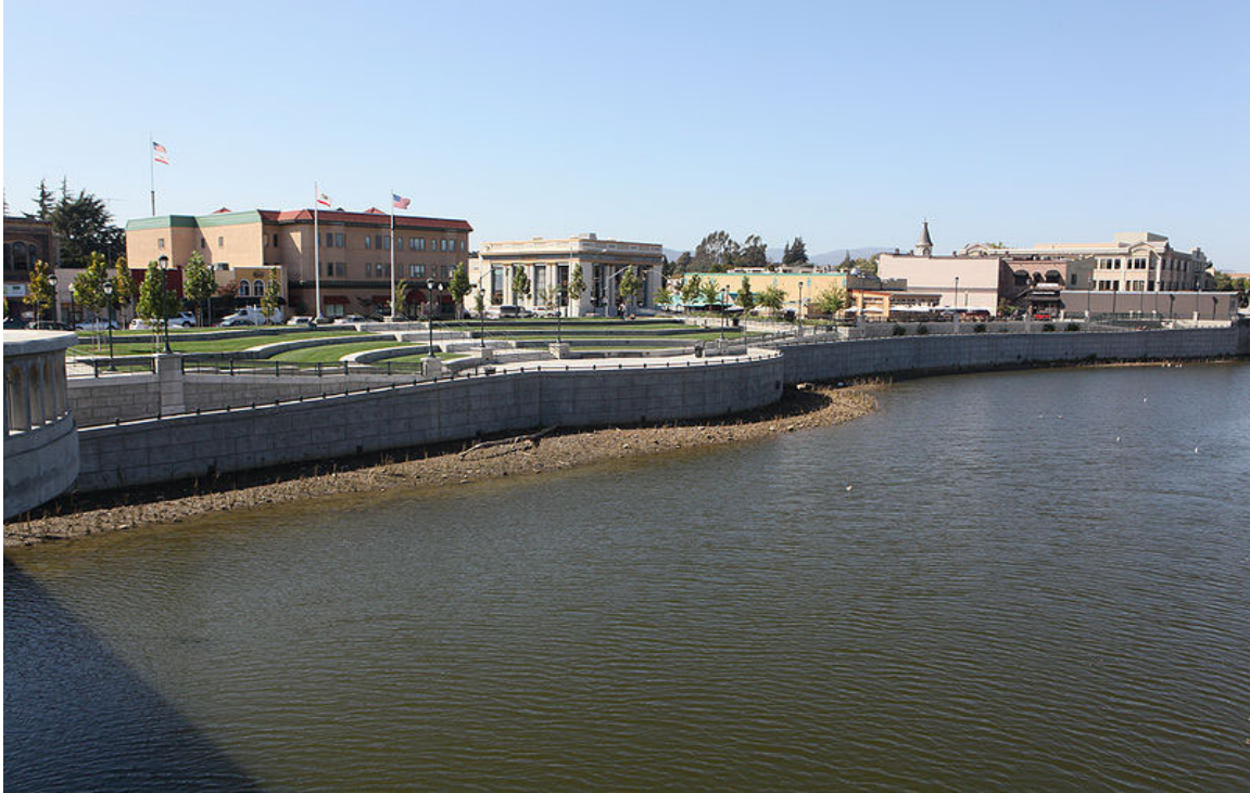
Figure 3-9: Example of floodwall
