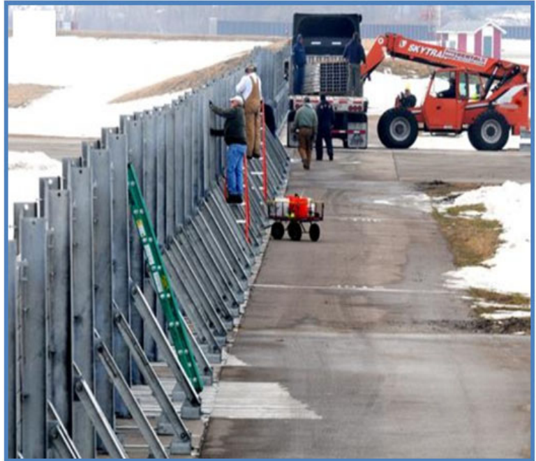
Figure 3-7: Installation of removable floodwall
